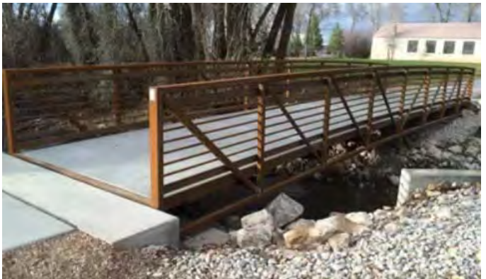
“Express” style pre-manufactured pedestrian bridge, CONTECH Bridge Solutions, a Continental Bridge brand
