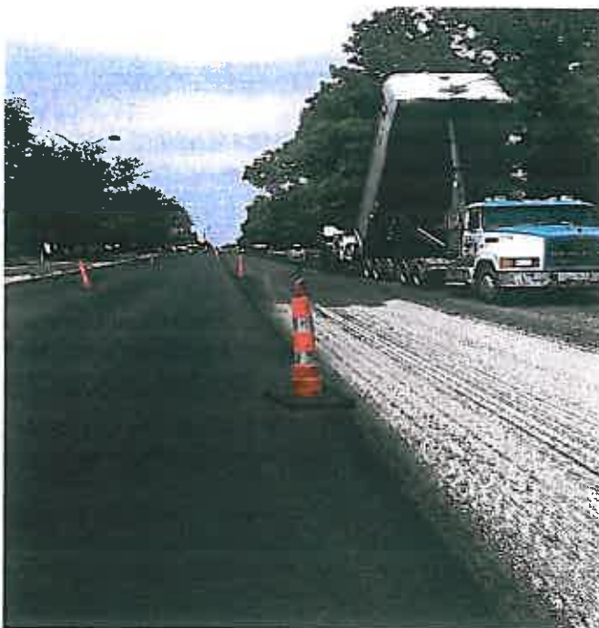
Second St. milling and overlay in progress
