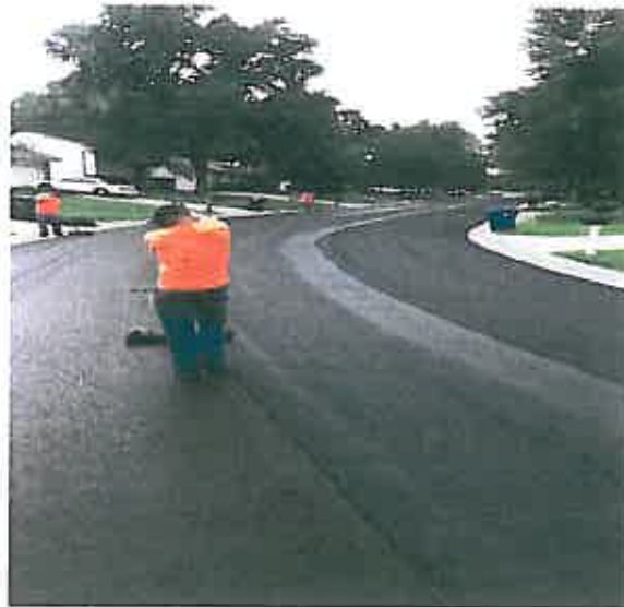
Slurry sealing process on Rockwood Blvd.
