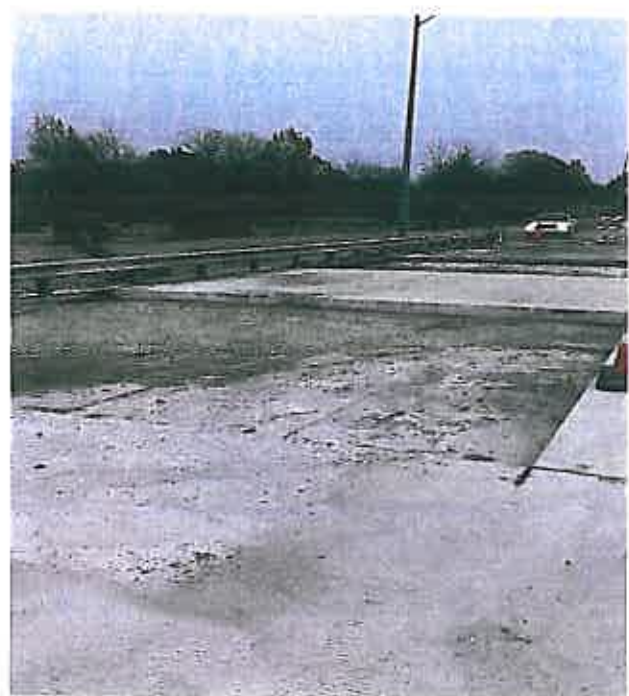
K-15 concrete panels removed for replacement
