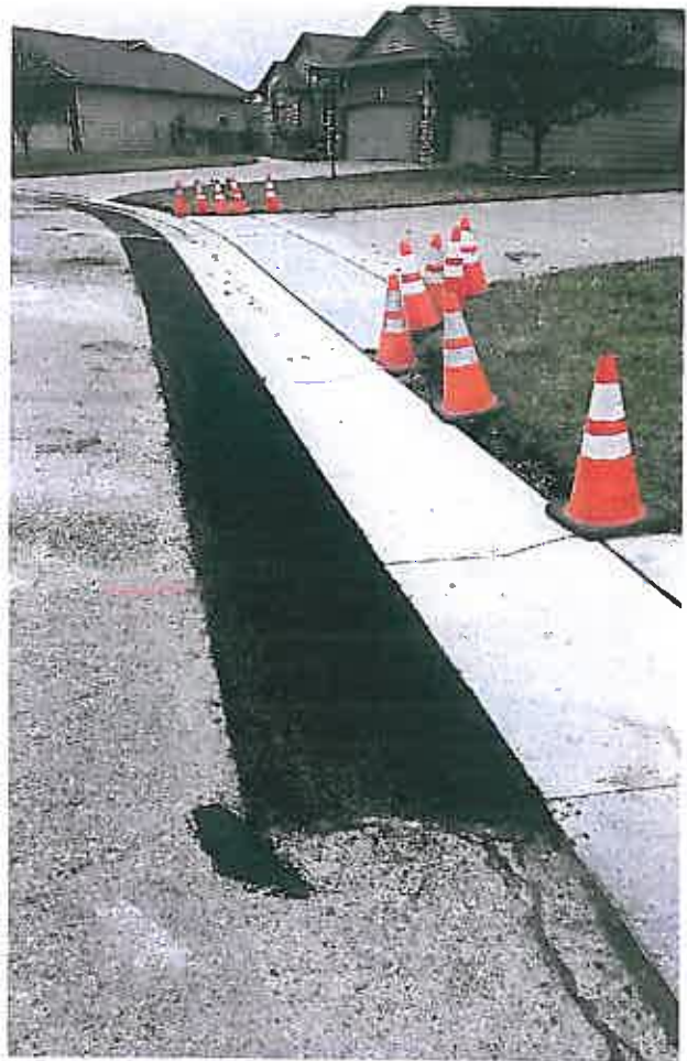
Curbing replacement on Fox Run Ct. - to eliminate significant pooling of standing water
