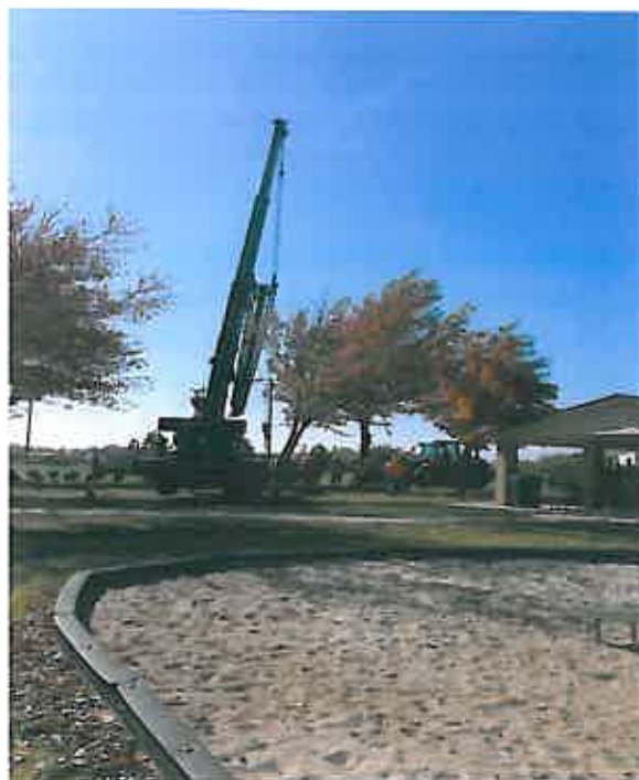
ROTTEN POLE BEING REPLACED BY CONCESSION AREA
