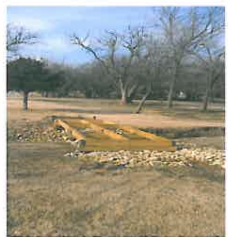
Large stone was put around the base frame of the new structure to combat erosion.
