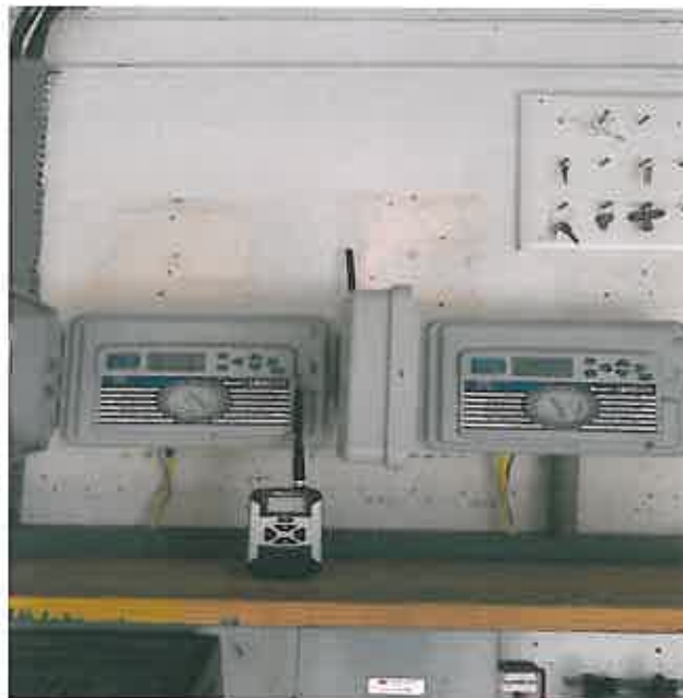
NEW CONTROLLERS INSTALLED, REMOTE READY
