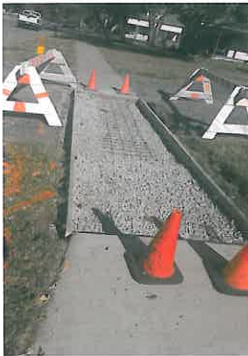
Sidewalk repair/replacement ready for cement
