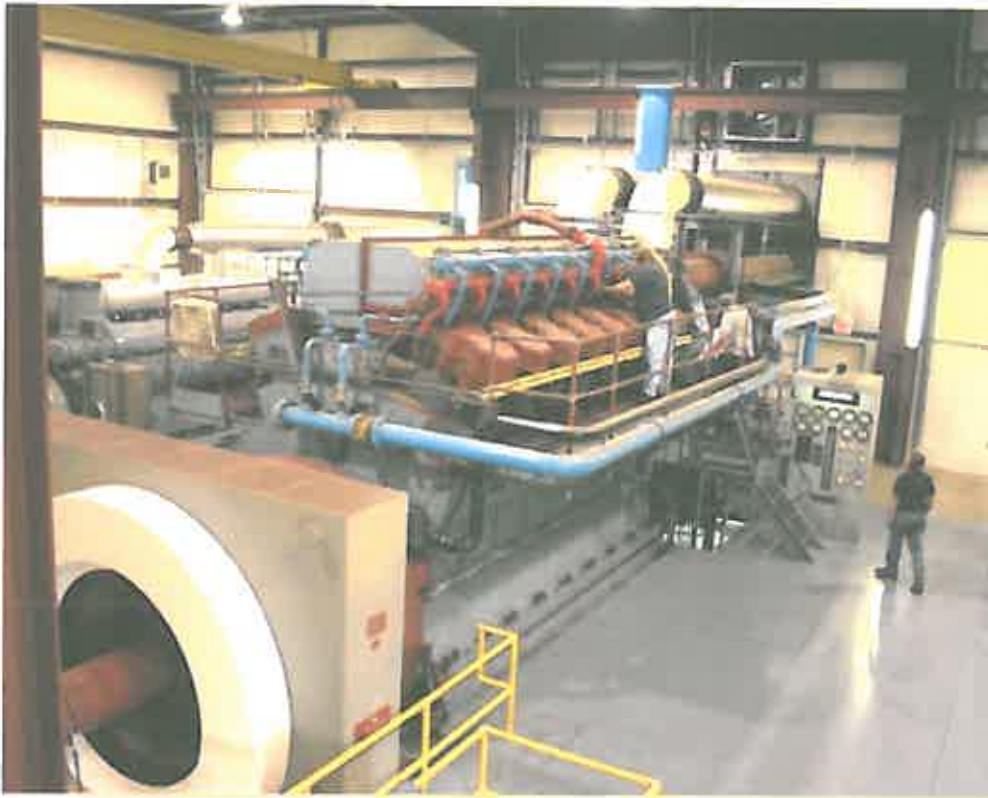
Above---Mulvane power plant staff are recording full load firing pressures on one of the three generating units located at the new power plant.
